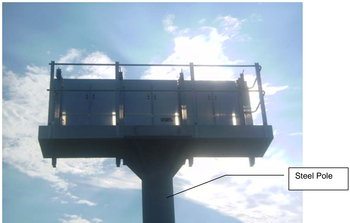
Rear Access DMS mounted on Aluminum pole
