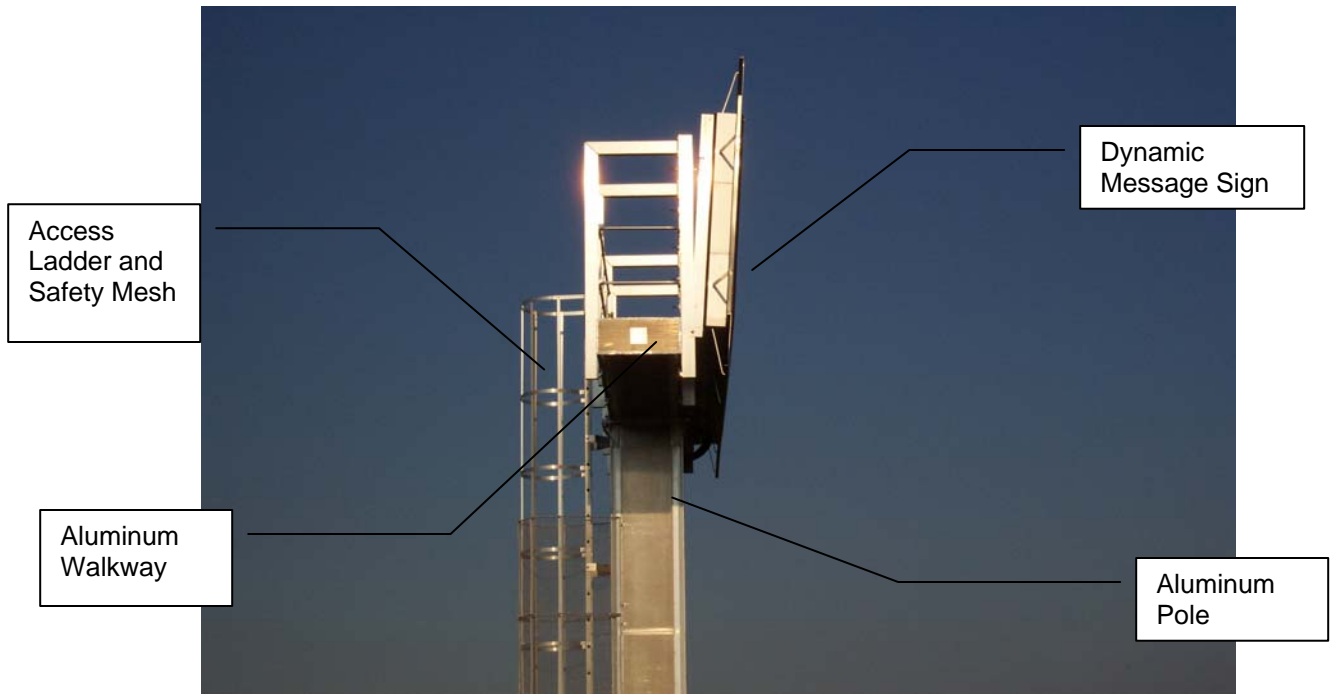
Rear Access DMS mounted on Aluminum pole
