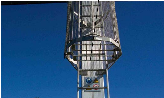
Ladder with Access Door shown in closed position
