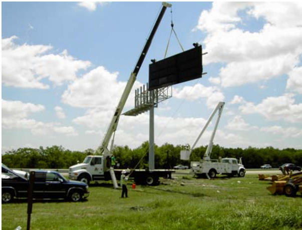
Assistance during installation
